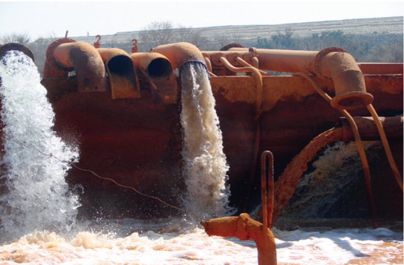
Figure 4.3: Water being pumped from the Eastern Basin to the treatment plant at Grootvlei Mine, before pumping ceased in 2011 27
